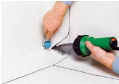
Close the bend on the vertical wall by spot-welding, pre-welding and welding.
