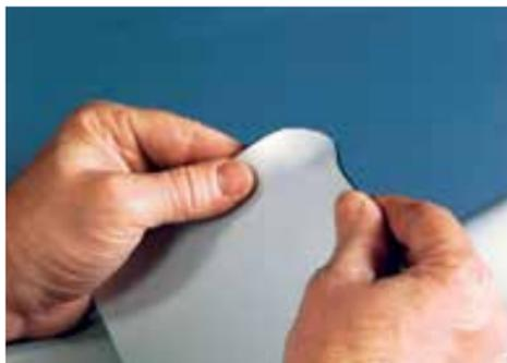
Round the corners of a square patch of TEXSALON TPO unreinforced membrane (*TEXSALON SA*) allowing a 2 cm excess for overlapping and welding. Heat and stretch the internal corner of the patch.
