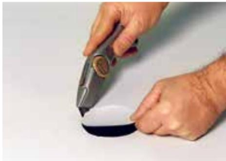
Only use outlets from the TEXSALON TPO range. Cut a hole in the roof membrane to correspond with the downpipe.
