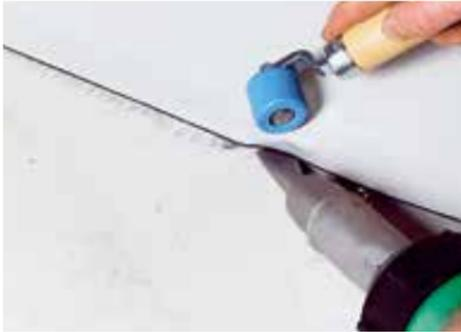
Re-align the new material. Spot-weld, pre-weld and weld to the existing membrane.
