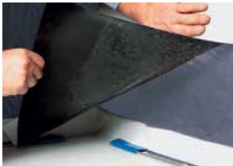
Bond the membrane to the upstand starting at the top edge and working down to the base.
