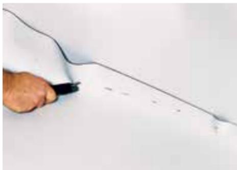
Install the TEXSALON field sheet. Bond and cut the membrane to form a bend of approximately 3 – 4 cm on the vertical wall. Once in position, cut the excess material to create a minimum upstand of 2 cm.
