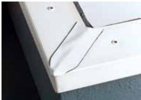
After positioning the neoprene or butyl sealing strip, mechanically fix the prepared flashing to the perimeter edge.
