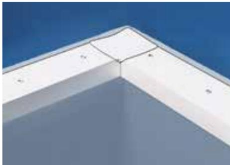
Spot-weld the flashing onto the profile starting 1 cm from the edge. The excess membrane from the vertical surface will form a pocket at the corner edge.
