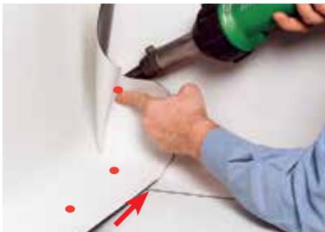
Cut and glue the second TEXSA flashing strip on the upstand, leaving 12 cm width for welding on to the horizontal surface.
