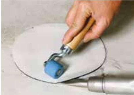
Spot-weld, pre-weld and weld the patch in place.
