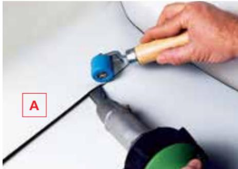
Spot-weld, pre-weld and weld the overlap on only the lower edge (A) of the horizontal surface.
